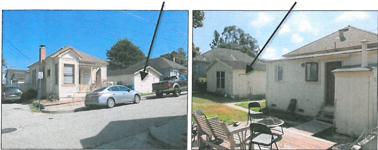
Figures 1 and 2. Left image shows the front (west) and left side (north) elevations of the house, with circa-1945 garage outbuilding at far right of image (arrow). Right image shows the rear (east) elevation of the house and garage (arrow).
