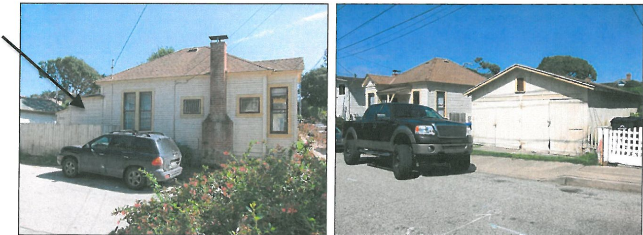
Figures 3 and 4. Left image shows the left side (north) elevation on Doc Ricketts Row with poorly constructed, circa-1926 rear addition shown with an arrow. Right image shows the circa-1945 garage outbuilding on 12 th Street.
